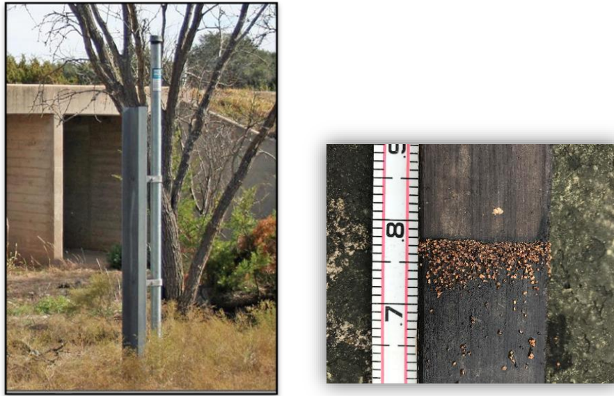
Figure 2.9 Photographs showing A, U.S. Geological Survey crest-stage gauge, looking downstream, and B, close-up of a typical enclosed wooden staff and cork line. The cork line marks the heights of a high-water mark during a flood event. Photographs by U.S. Geological Survey.
