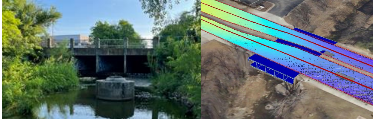
Figure 35 3D culvert model for a bridge-class culvert on Anderson Lane at Shoal Creek in Austin, Texas.
